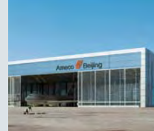
Ameco A380 Hangar Peking, China
